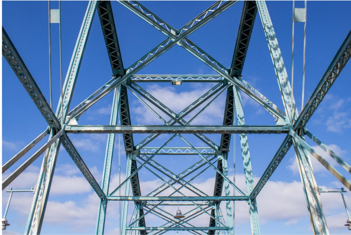
"Trusses." Derek Bruff, Flickr (C)
